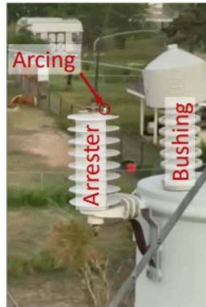
Figure 2. Falling jumper, arcing but providing service, without customer complaint (case study 1)
