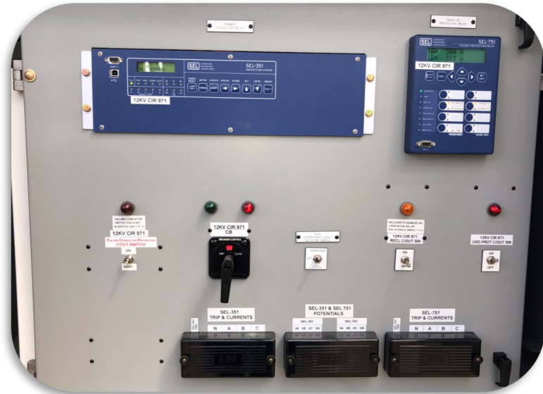
Circuit Breaker Controls, Enable Light & Switch
