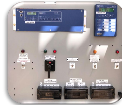
Digital Relay Equipment
