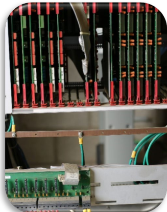
Aging Remote Terminal Units
