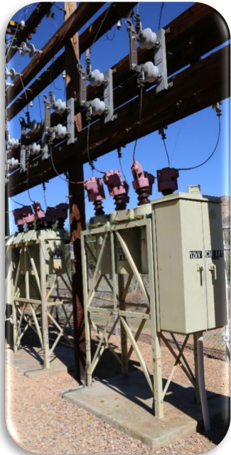
Oil Circuit Breakers
