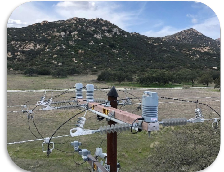
Line Monitor Sensor
