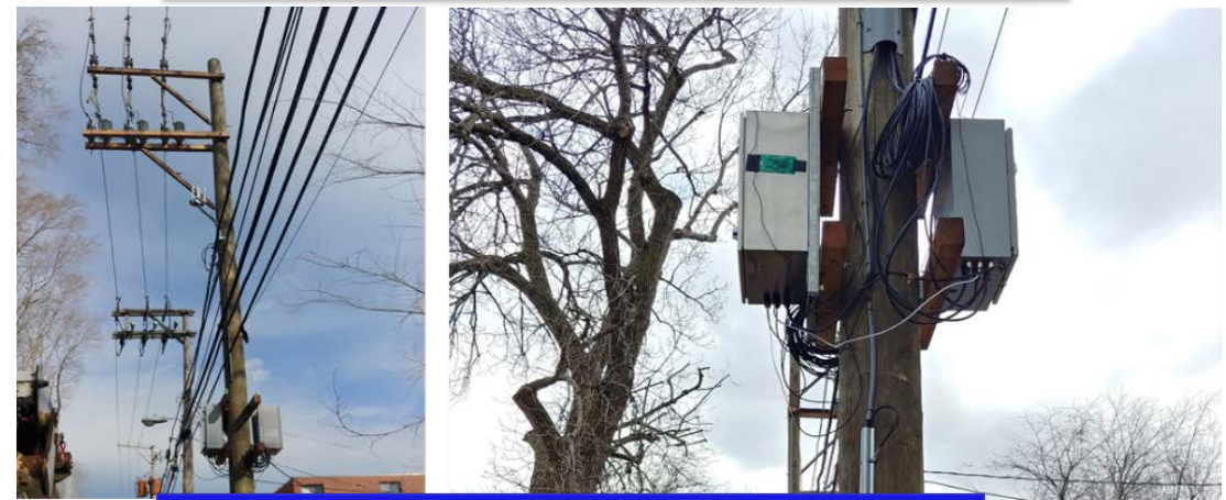
SIMPLE 2 and MVCAL Cabinet
