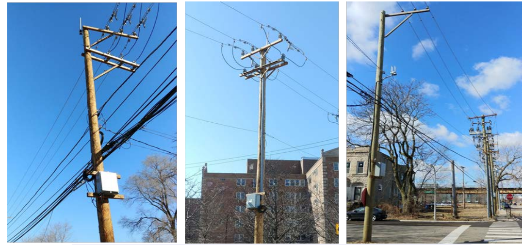
SIMPLE 1, SIMPLE 3 and the POI cabinet
