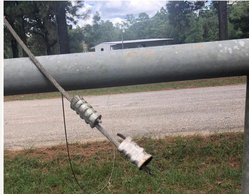
Conductor burn-through at clamp
