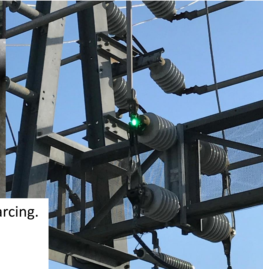
Substation blade switch
