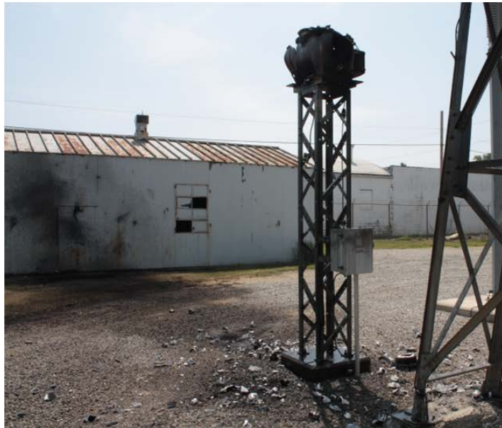
Example of failing CCVT in a substation
