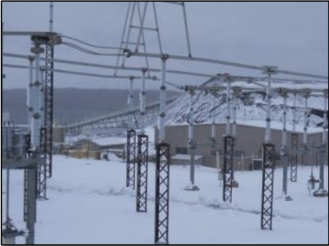
Use of resistive glazed insulators or stepped shed designs
