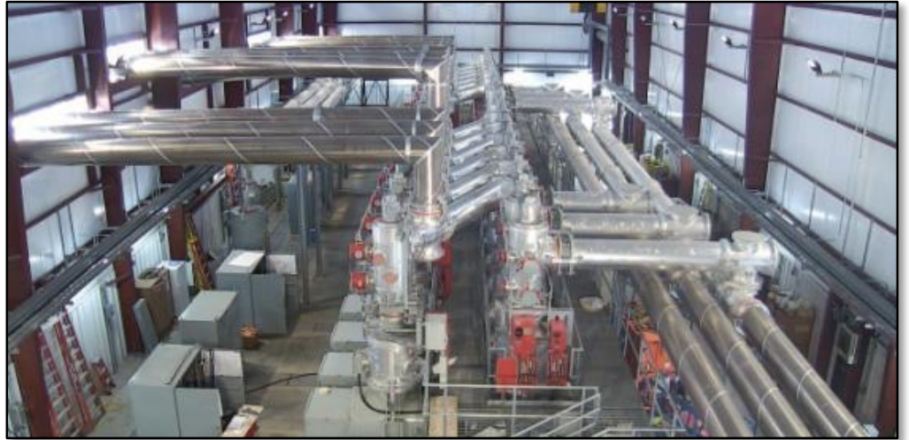
Gas insulated switchgear mounted indoors
