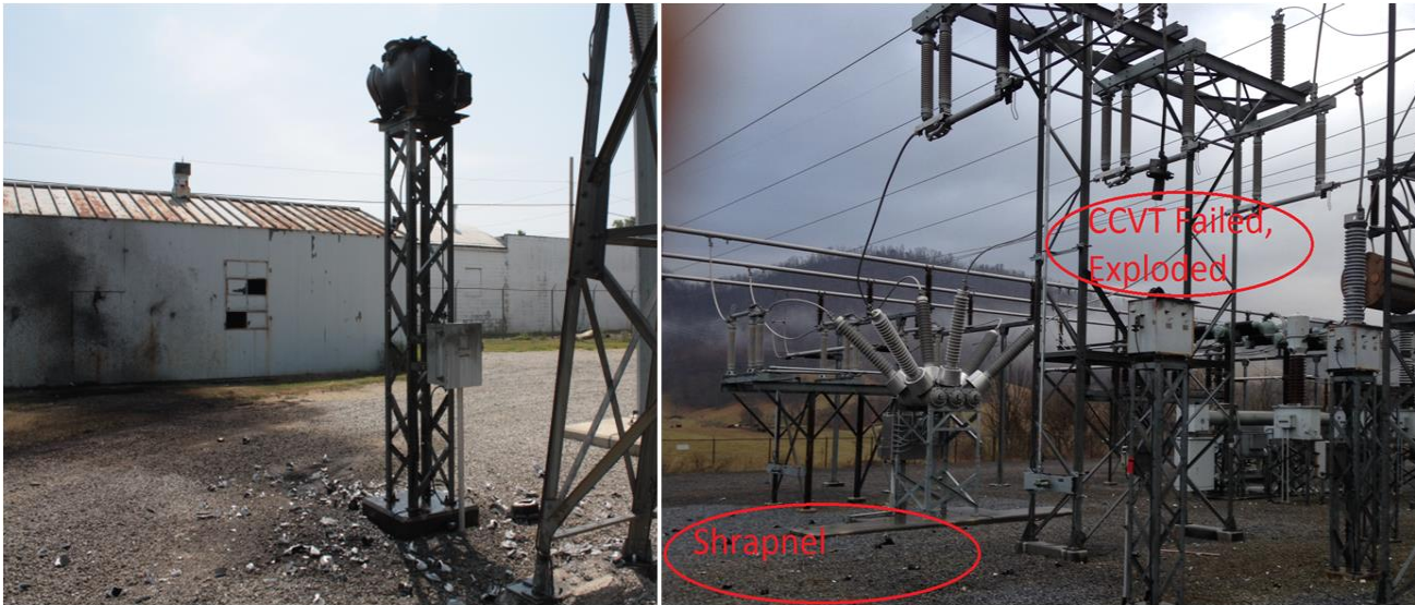
Example of failing CCVT in a substation
