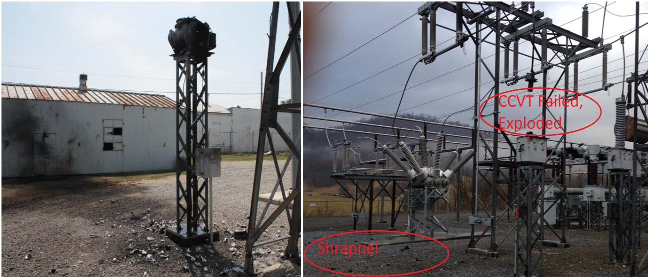
Example of failing CCVT in a substation
