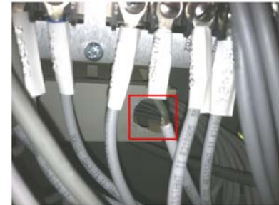
Open Circuit in CT secondary due to Wiring damage
