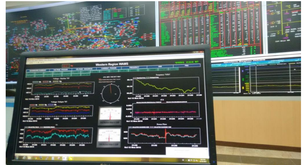
Synchronization Display at Control Centre
