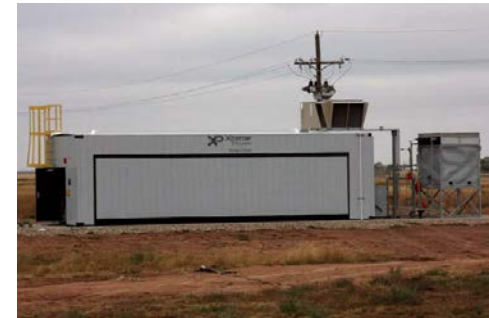
CCET provided a 1 MW utility scale battery system at Reese Technology Center.
