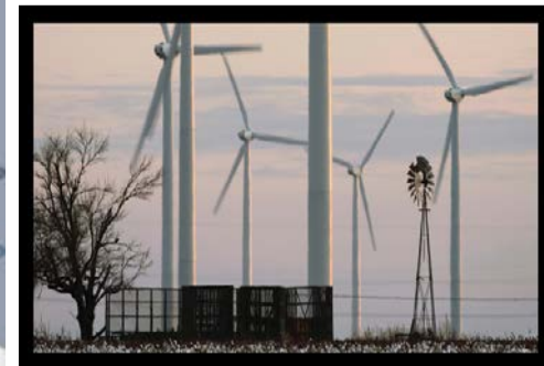
Reese Technology Center had six wind turbines operating in 2013.
