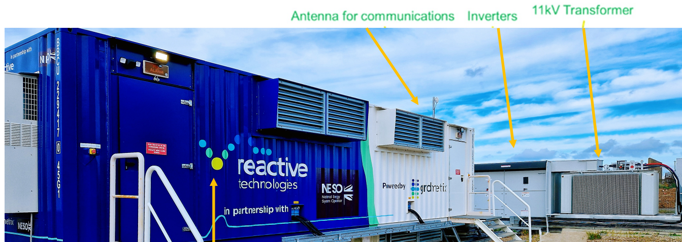
Container houses ultracapacitor cells and modules, control system, cooling system, fire detection and suppression
