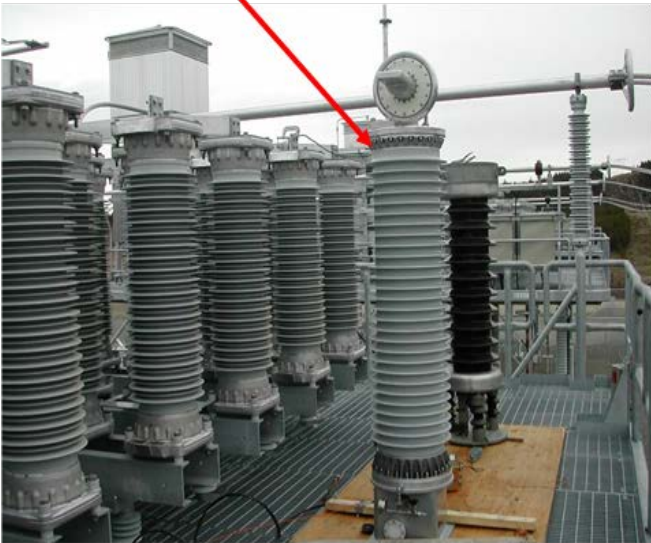
MOV Voltage Measurement
