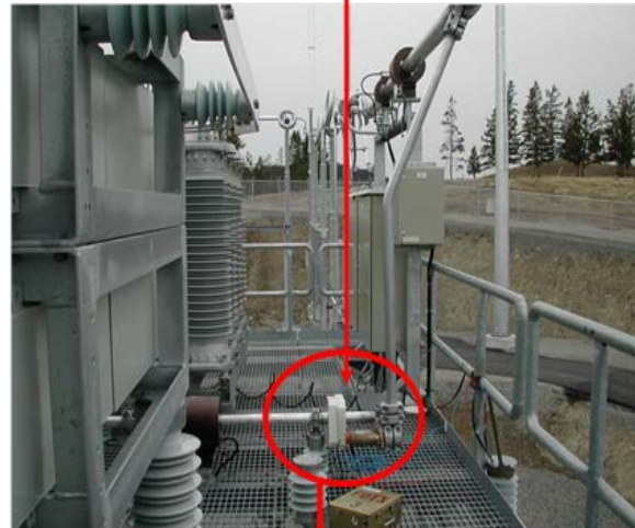
MOV Current Measurement
