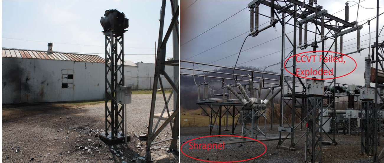
Example of failing CCVT in a substation
