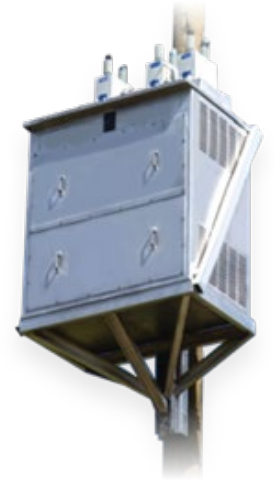
PQ Correction Equipment (Harmonic Filters & Capacitor Banks)
