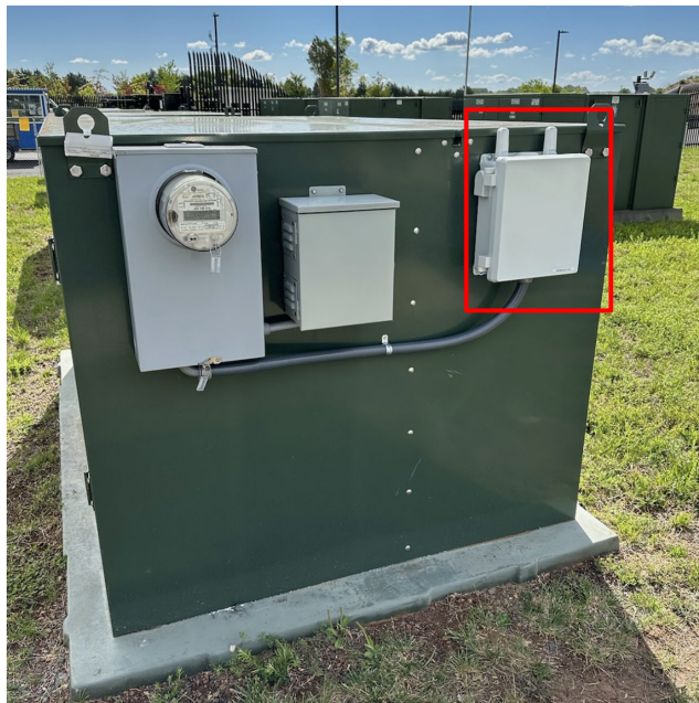
PQube 3 PQ Monitor Data Center Installation
