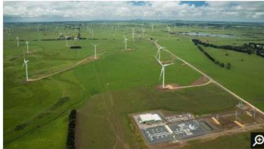
Vestas turbines and power plant control.
