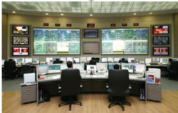
System Control Center
